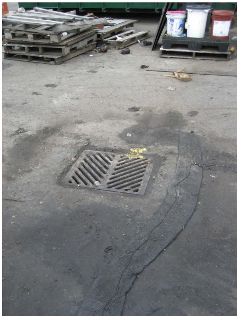
Photo 3: A catch basin on the northern portion of the ConGlobal Industries container terminal located near the maintenance area (eastern parcel).
