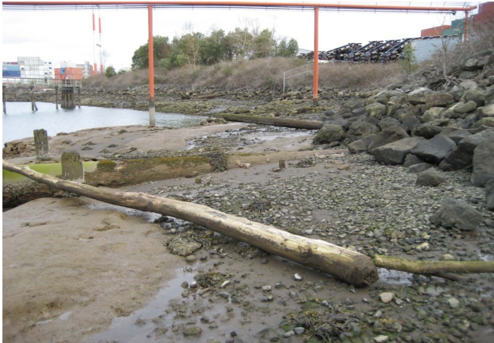
Photo 15: View (looking north) of the north-central and northern portions of the T-108 shoreline; the bank in this area is armored with rip-rap.
